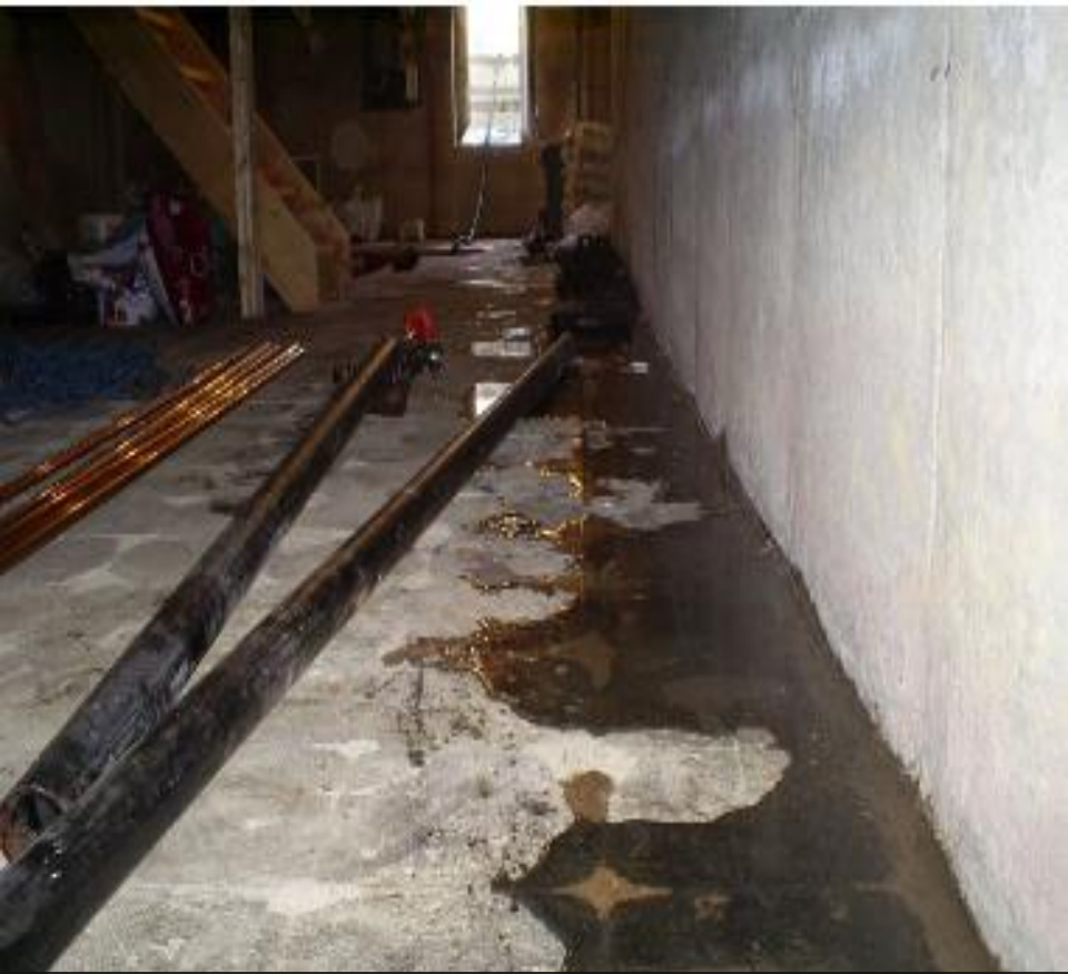
Delaminated under the membrane. Leaking at a cold joint. Both already past the barrier.
