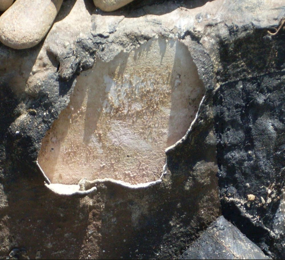
Delaminated under the membrane. Leaking at a cold joint. Both already past the barrier.
