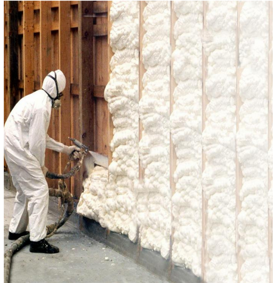
ocSPF must be scarfed and supported
