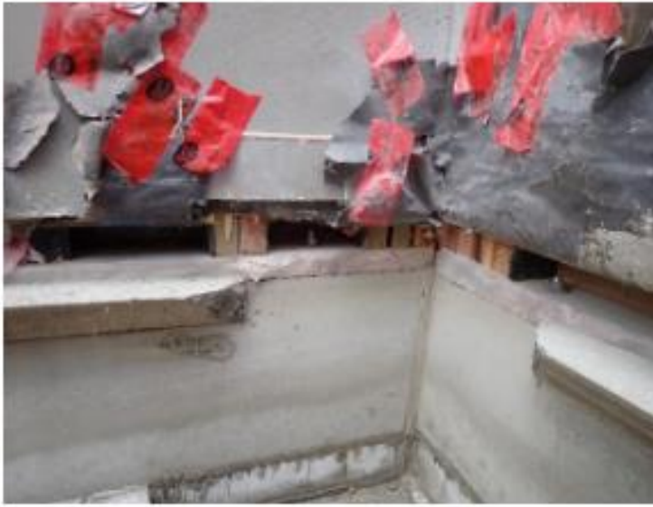
New conc. curb
