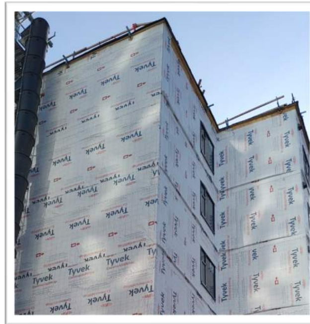
LOOSE-LAID SHEATHING MEMBRANE APPROACH
