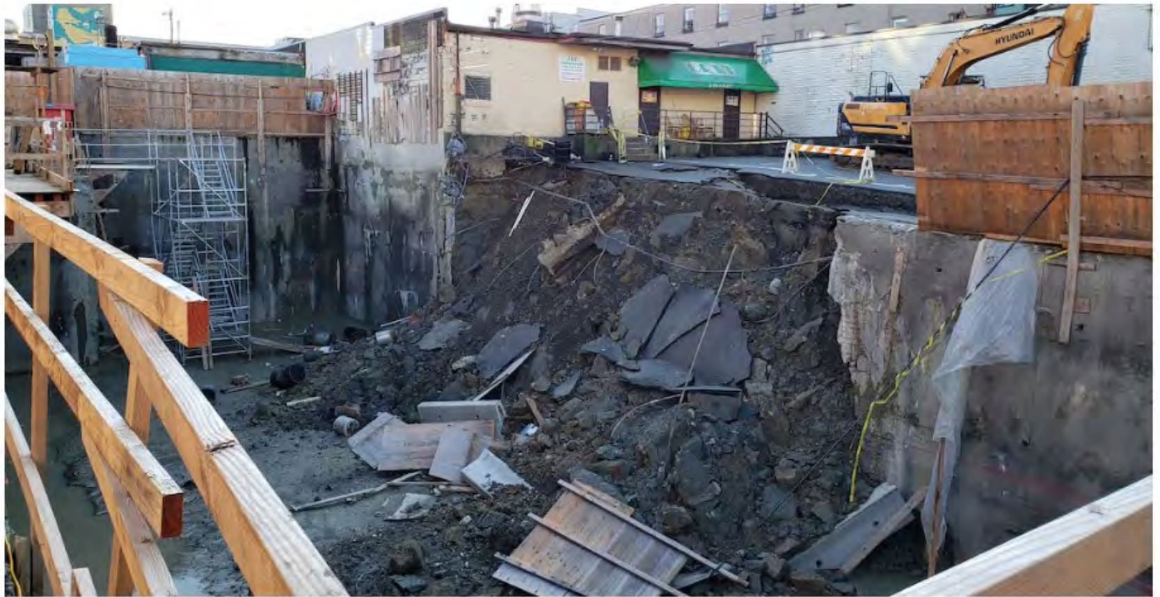
Site of the construction pit collapse at 138 East 8th Avenue, Vancouver. (Kenneth Chan / Daily Hive)
