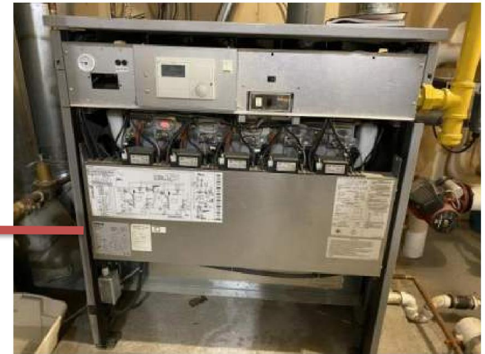
Boiler: AERCO MLX757H Condensing 92% E t
