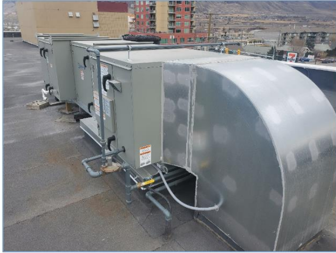
Corridor MUA: Gas fired (3120cfm)
