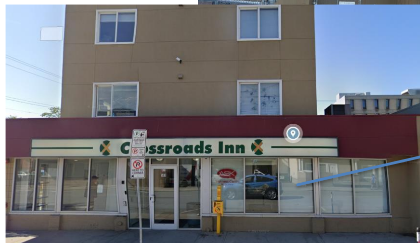
Storefront windows: Aluminum, non-thermally broken, double glazed (U1.1 SHGC 0.8) Original (1993)
