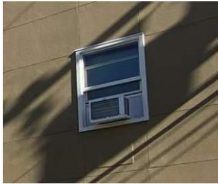
Cooling: Window mounted AC
