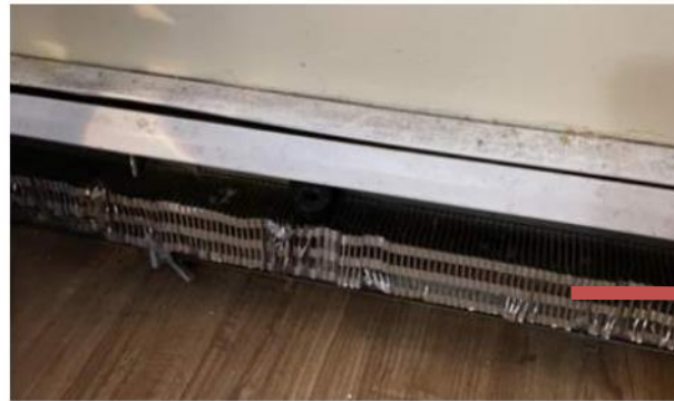
Heating: Hydronic baseboard heater
