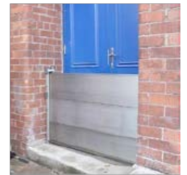
Figure 2 Demountable type barrier on external door 2 donated by www.lakesidefloodsolutions.co.uk
