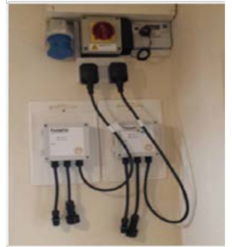
Figure 1 Sump pump controls are on separate circuit, fixed high above water level
