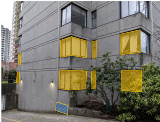
UNPROTECTED OPENINGS NEAR EXTERIOR EGRESS FACILITIES AT EAST ELEVATION
