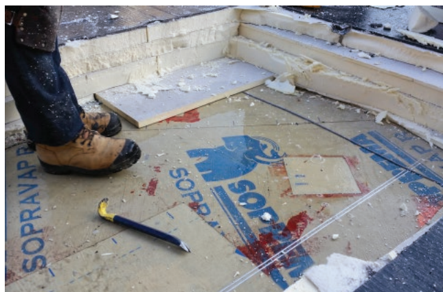
SMT STAINLESS STEEL MOISTURE DETECTION TAPE INSTALLED UNDER ROOF MEMBRANE REPORTS ON STATUS OF MOISTURE CONTENT, IN THIS CASE WATER INTRUSION FROM TEMPORARY NIGHT SEAL.
