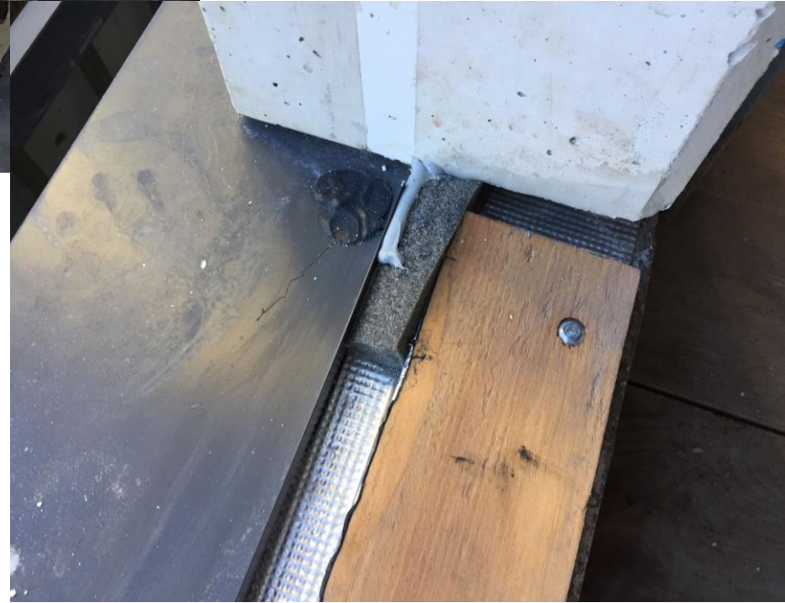
CONC UPSTAND CURB @ LVL 4 NORTH FACADE; PRECAST INTERFACE
