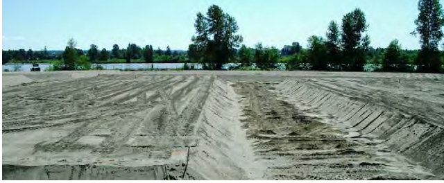
Photo 6: Example of preload in place on a future building site.
