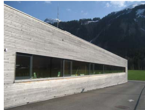
CanPHI fire station
