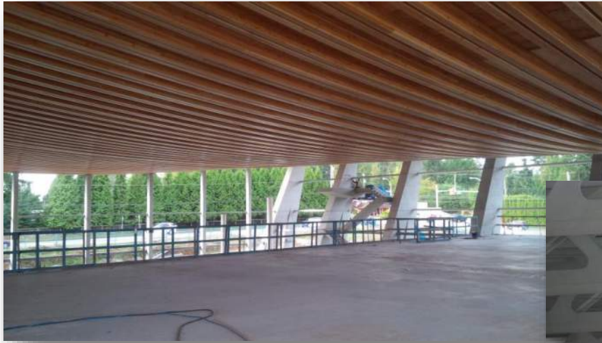
Structural Wood Roof Deck, Concrete Walls and Columns
