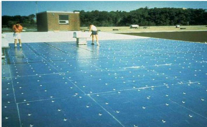
**100 squares of 4 x 8 foot board material has more than a half mile (3,650 linear feet) of board joints!**
