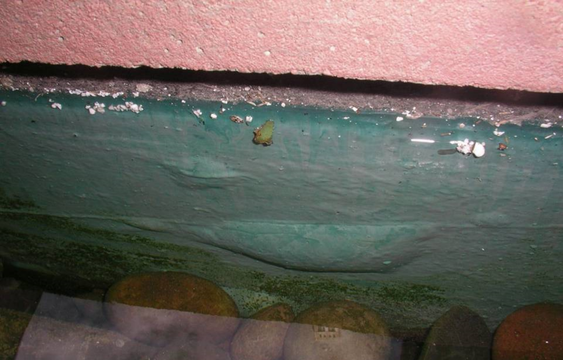
Water Filled Blisters in Water Features
