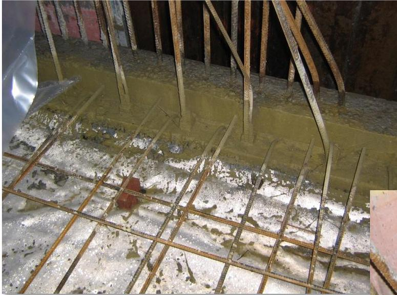
**Slurry applied to pony wall transition prior to pouring slab on grade**
