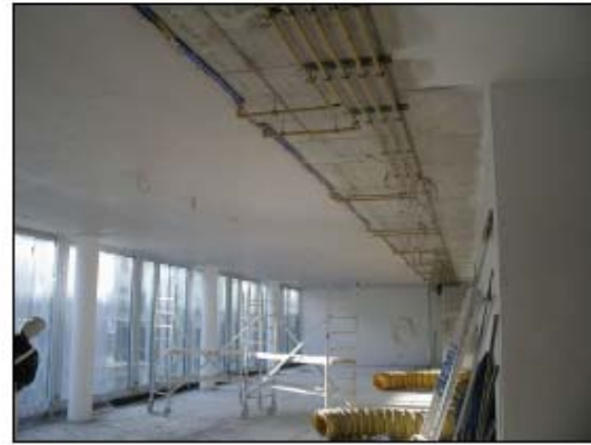
PLASTER APPLIED OVER MATS – HEADER CONNECTION TO DISTRIBUTION PIPING
