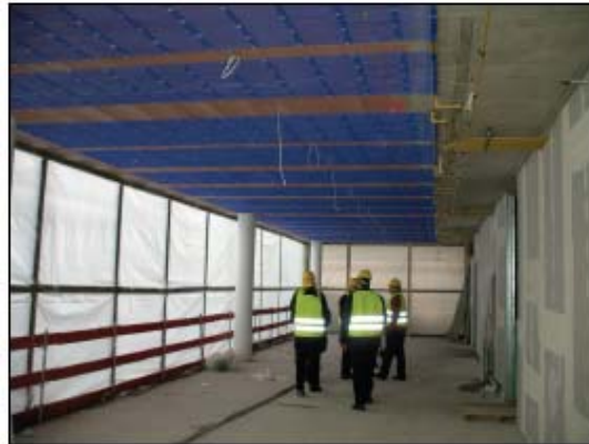
MATS READY FOR PLASTER. HEADERS IN CORRIDOR
