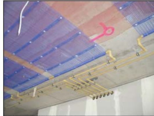
MAT HEADERS ROUTED TO CONTROL CENTRE
