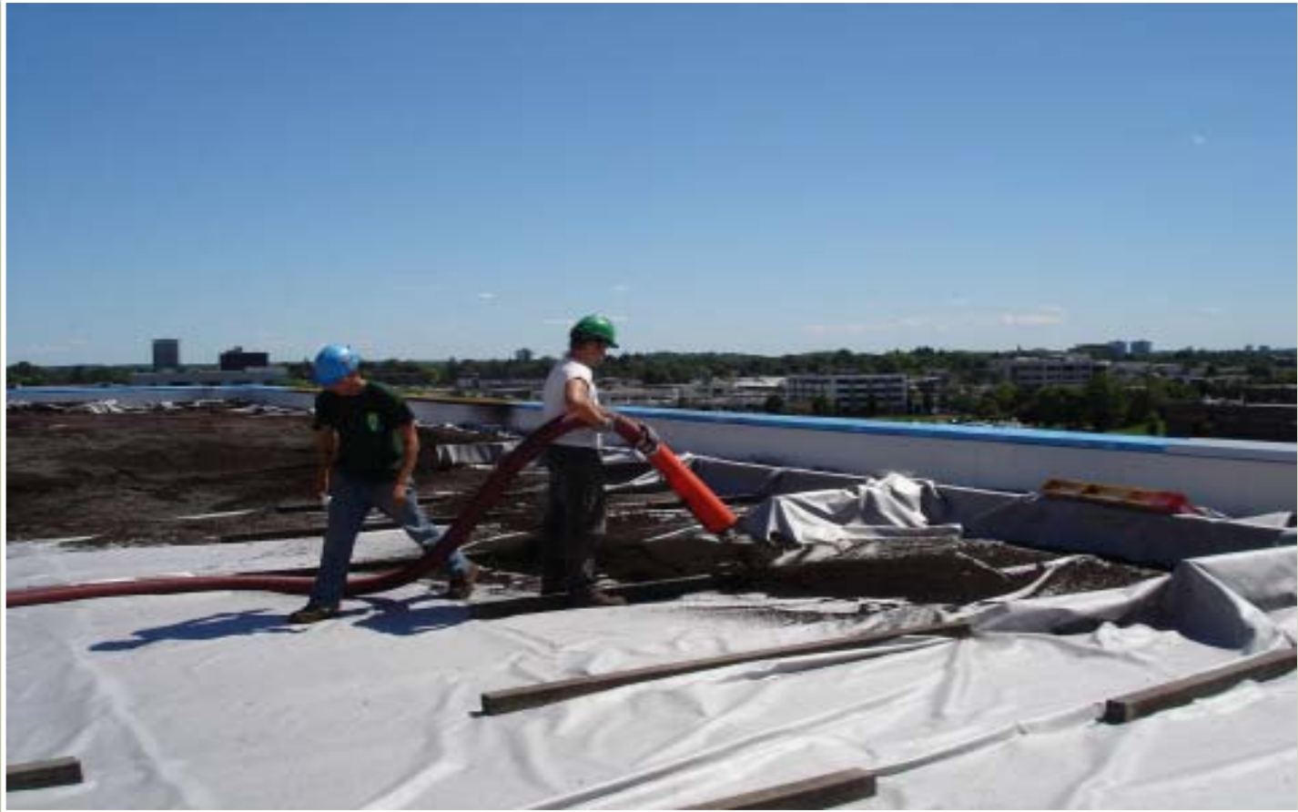
Soil is blown onto roof (Source: HydroTech)
