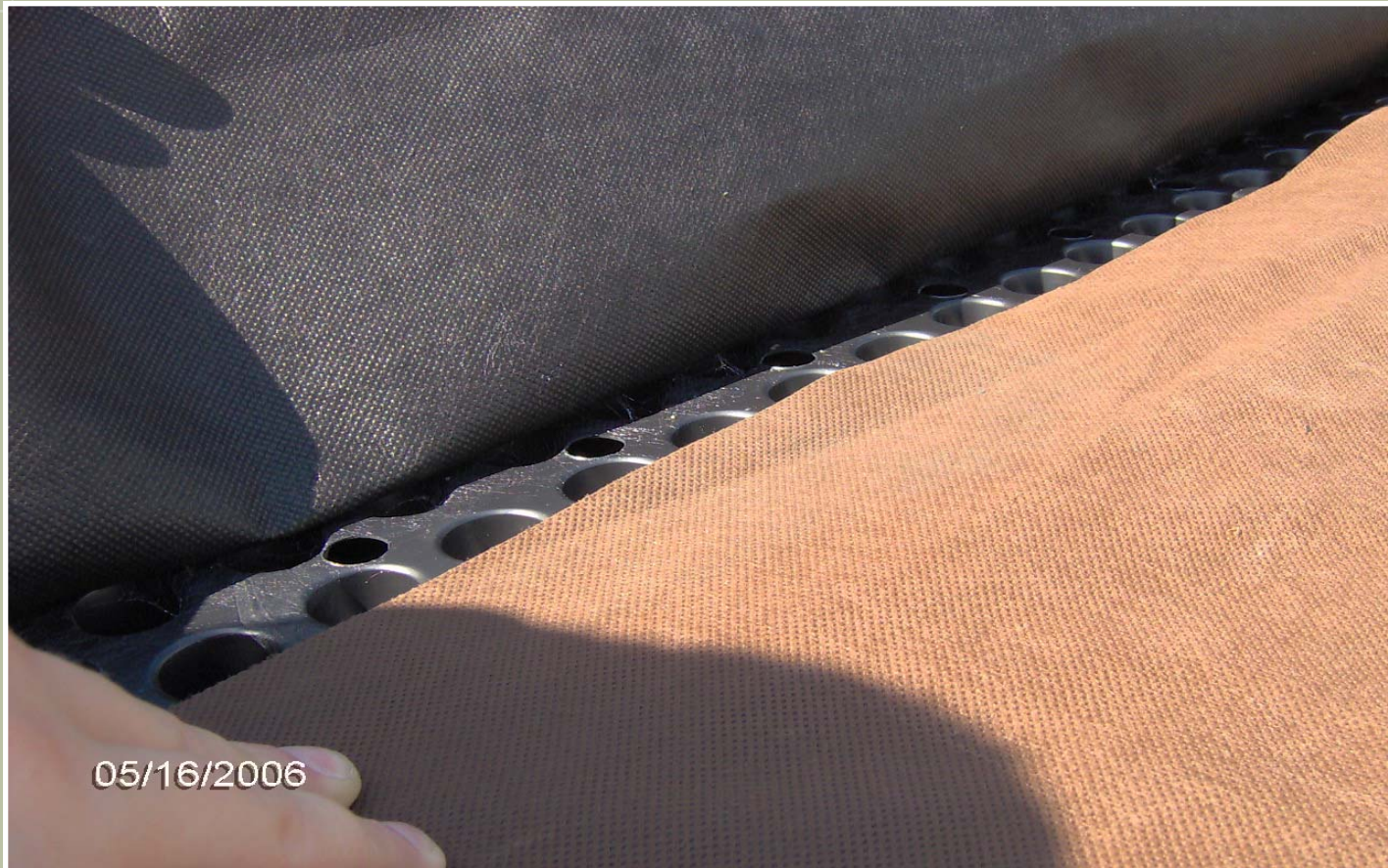
Root barrier chemical treated filter cloth
