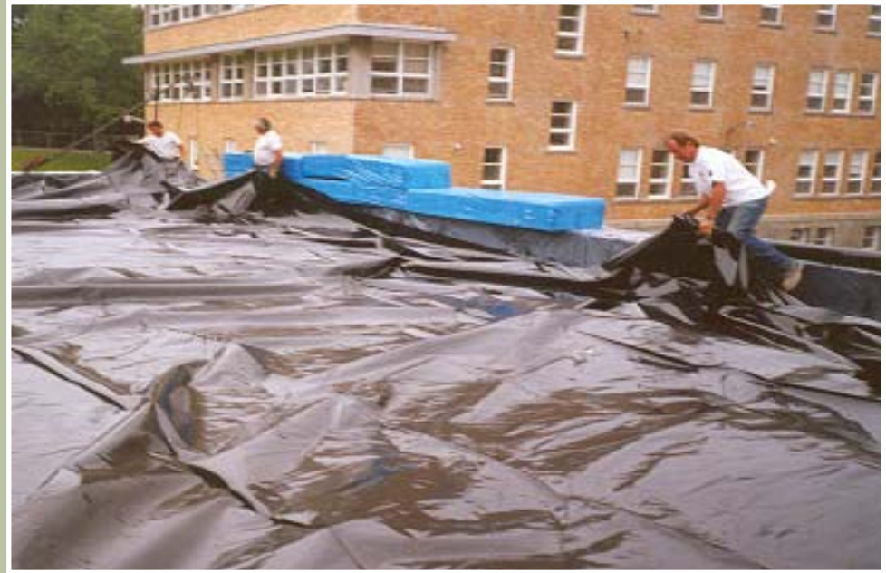
Root barrier and installation (Source: HydroTech)
