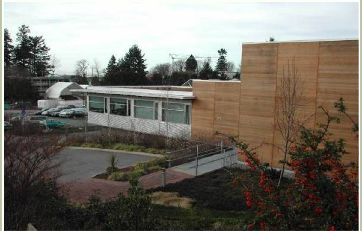
City of White Rock Operations Building, White Rock, BC
