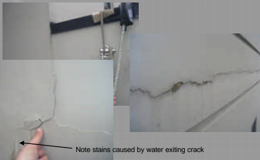
Case Study 2 – No crack control planning = Cracks everywhere
