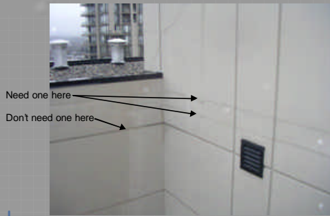
Case Study 2 – Inadequate Location for Architectural reveals
