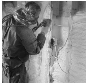
Figure 13: ½-pound spray foam application
