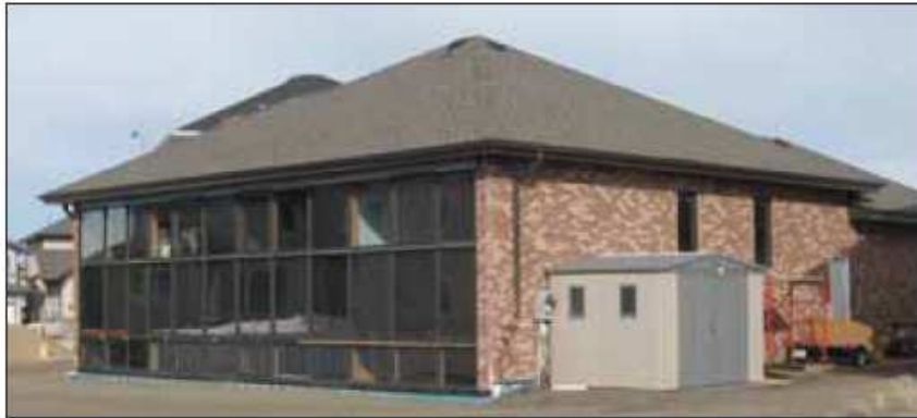
Figure 1 The Factor 9 Home viewed from the south east. The view is of the back side of the house. The solar thermal panels (1.5 metres tall) are in a horizontal band between the upper and lower windows.
