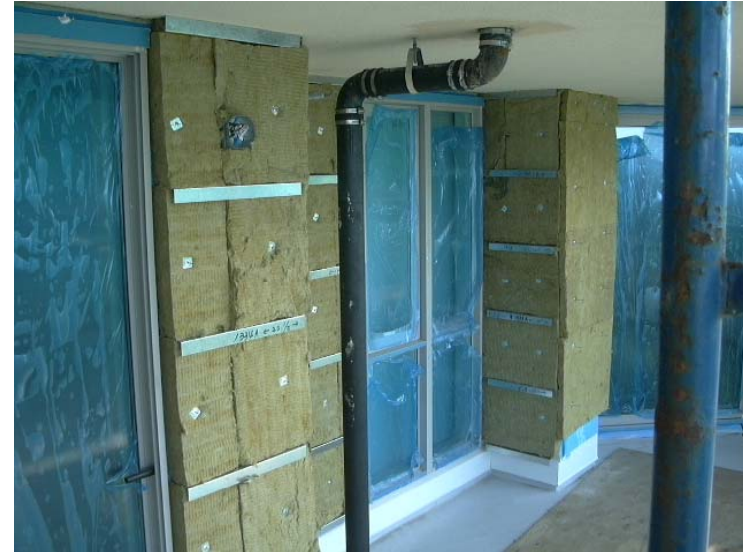
Cladding Girts Metal Panel Wall
