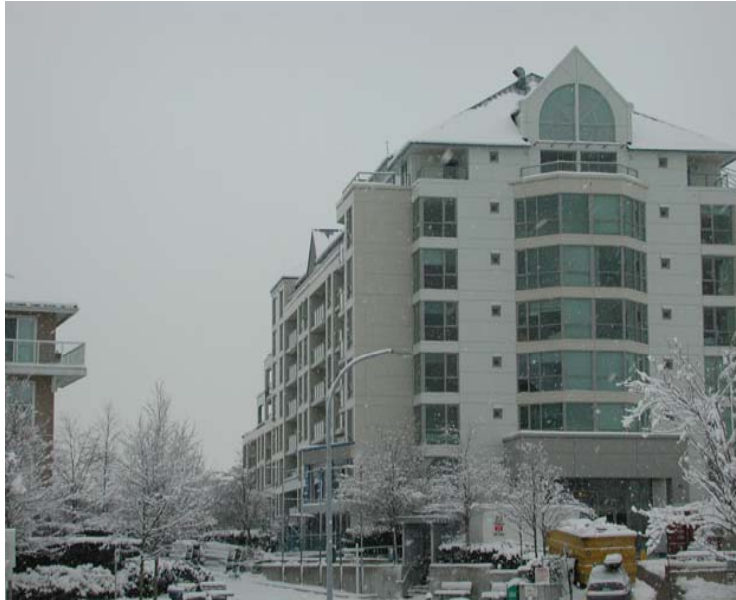
Steel Stud & Metal Panel Wall
