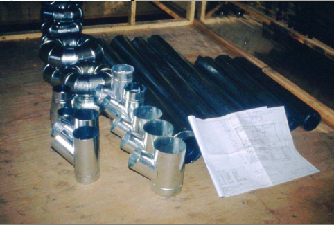
Good Material, potentially Good installation
