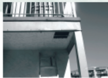
Paint peeling from a metal flashing: Good quality factory-finished metals would have better endurance than this site-painted metal flashing.
