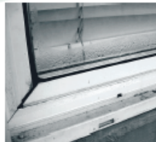
Condensation forms first on the coldest surfaces of a room, usually on glass surfaces of windows and doors.
