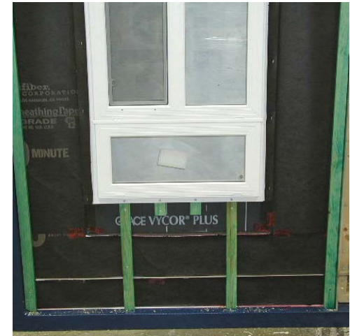
Window installed over furring strips
