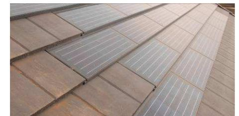
Photovoltaic roofing tiles
