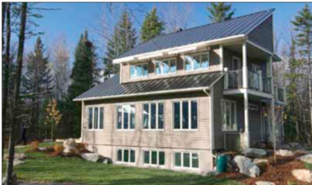
Figures 7 and 8 ÉcoTerra™, an EQuilibrium™ demonstration home in Eastman, Quebec uses amorphous PV panels stuck directly on its metal roof
