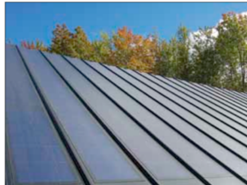
Figures 7 and 8 ÉcoTerra™, an EQuilibrium™ demonstration home in Eastman, Quebec uses amorphous PV panels stuck directly on its metal roof
