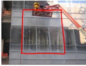
Figure 17: Identification of representative area for field testing (metal and glass curtain wall).
