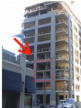
Figure 14, 15 and 16: Identification of representative areas for field testing (precast concrete / punch window wall assembly).
