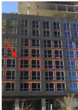
Figure 14, 15 and 16: Identification of representative areas for field testing (precast concrete / punch window wall assembly).
