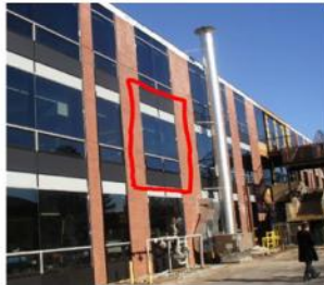
Figure 18: Identification of representative area for field testing (metal and glass curtain wall and adjacent masonry assembly).
