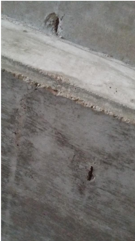
Concrete spalling
