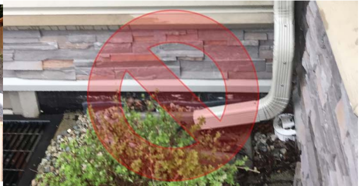
Photo 6: Example of a very poor drainage system: rainwater downspout drains to a splash pad which directs water towards building foundation wall and adjacent to poor building enclosure membrane termination
