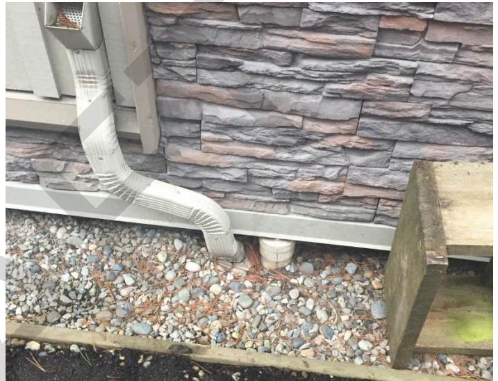
Photo 12: Cleanout is blocked by the building and not accessible.
