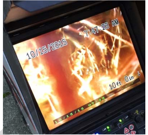
Photo 16: A foundation drainage pipe overgrown with roots.
