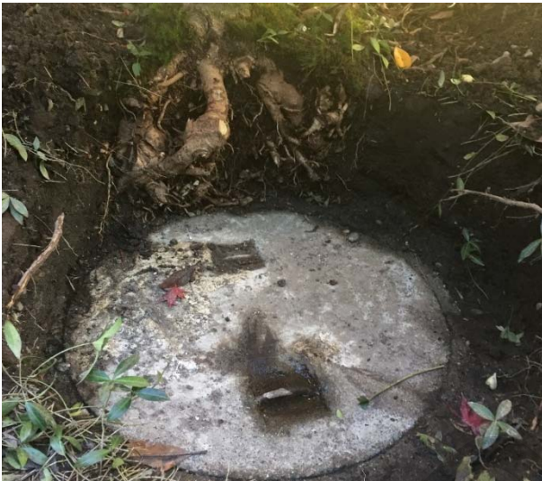
Photo 11: Building sump at a building found buried in the garden area and noted to be full of sediment and vegetation.
