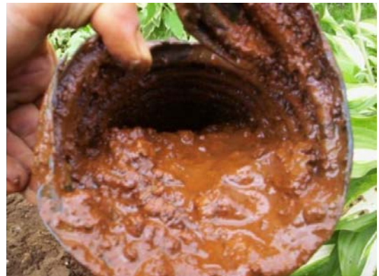
Photo 13: Example of iron ochre clogging a pipe.
