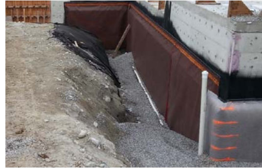
Figure 9: Typical best practice detail for a foundation drainage system. Photo 3: Perimeter drainage on building with gravel bedding.
