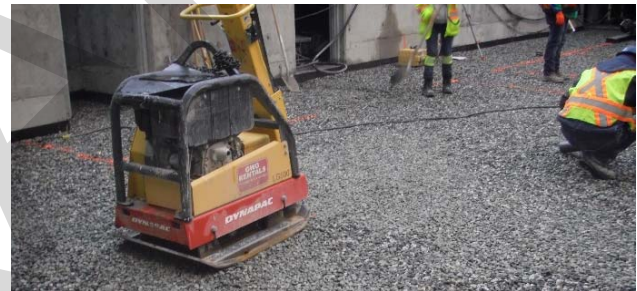
Photo 1: Example of clear crushed gravel being placed and compacted for underslab drainage.
