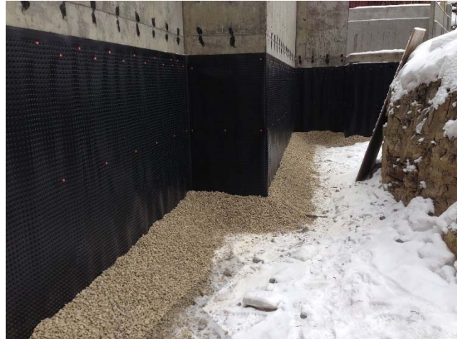
Photo 4: Typical drainage membrane installation.
