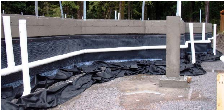
Photo 5: Example of a well-constructed foundation drainage system: drainage membrane applied over the damp-proofing agent, PVC foundation drain pipes have been bedded in clear gravel wrapped in filter cloth, rainwater leader downspouts directed shallow solid pipes.
