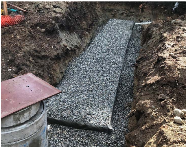
Photo 9: Example of an infiltration tank.
