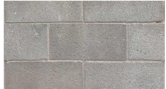
Most CMU is not an airtight material by code definition unless coated
