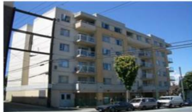
The residential building for indoor climate testing in Vancouver
